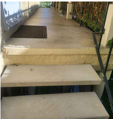
Walkway: *Walkway Inspection Image(s)
