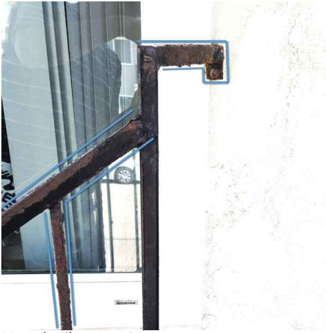
Handrail corrosion
