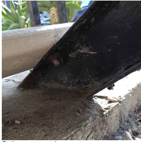
Stringer corrosion
