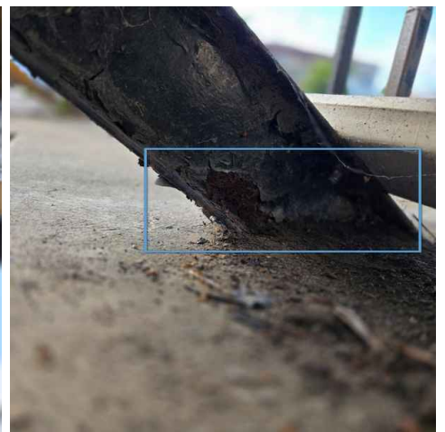
Stringer corrosion
