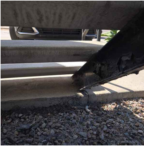
Stringer corrosion
