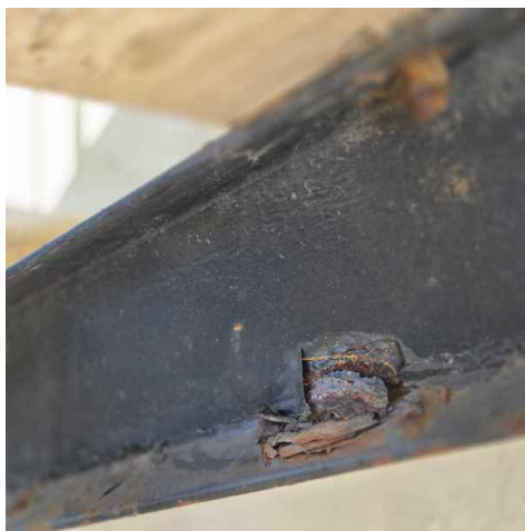
Stringer corrosion
