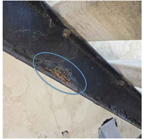
Stringer corrosion
