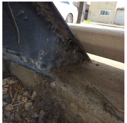
Stringer corrosion
