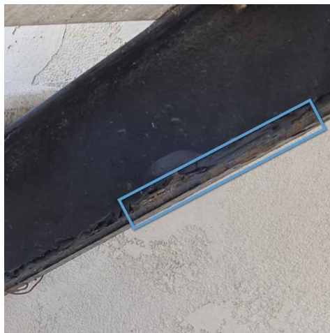
Stringer corrosion
