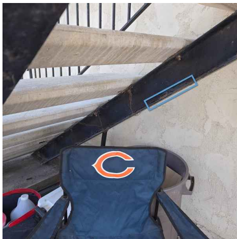
Stringer corrosion
