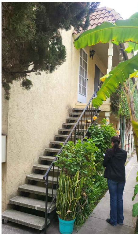
Stairs to walkway
