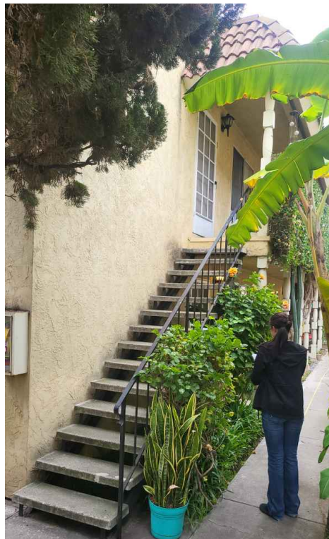
View of stairs and walkway E3s
