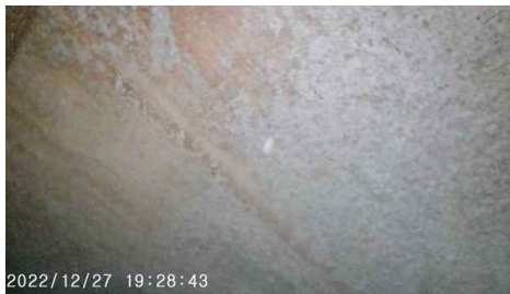
Crack across concrete deck
