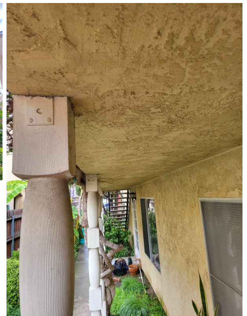
Underside of walkway S view
