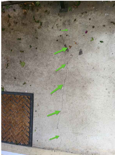
Crack across concrete deck
