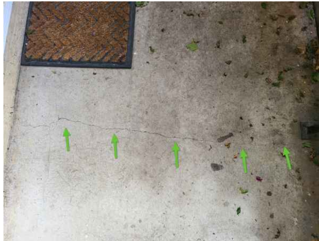
Crack across concrete deck
