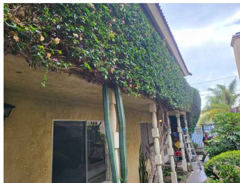
Underside of walkway N view
