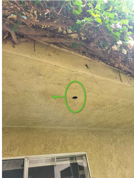
1st borescope inspection
