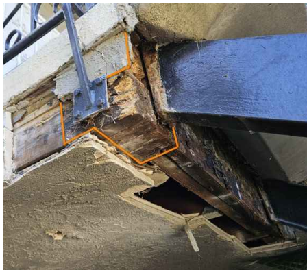
rotten joist
