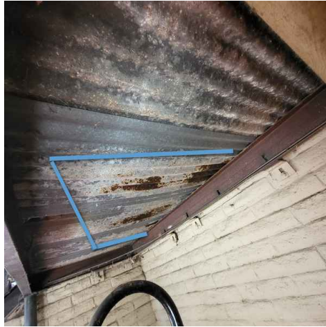
Underneath Landing Walking Structure
