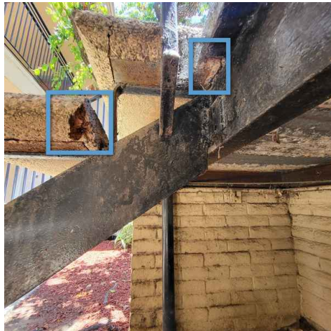
Thread shows severe aging
