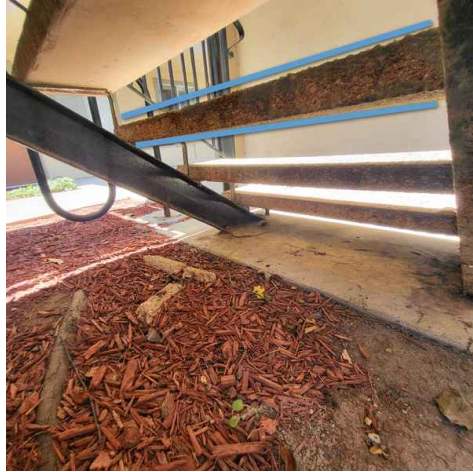
Thread shows severe aging
