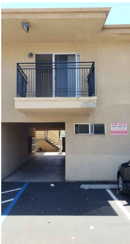
Apt. 30 Balcony : *Balcony Inspection Image(s)
