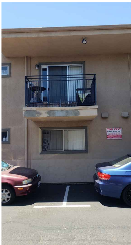
Apt. 16 Balcony : *Balcony Inspection Image(s)
