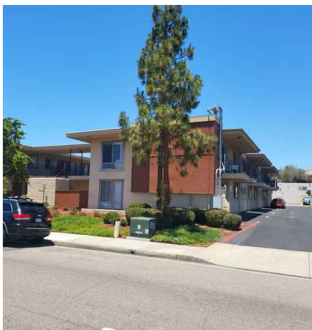
Apt. 8 Balcony : *Balcony Inspection Image(s)
