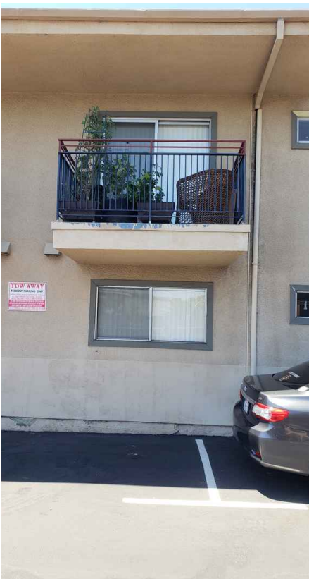
Apt. 10 Balcony : *Balcony Inspection Image(s)
