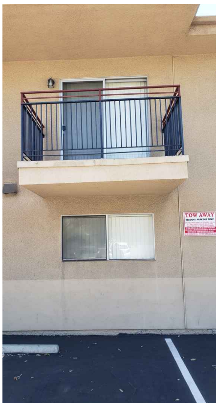
Apt. 36 Balcony : *Balcony Inspection Image(s)
