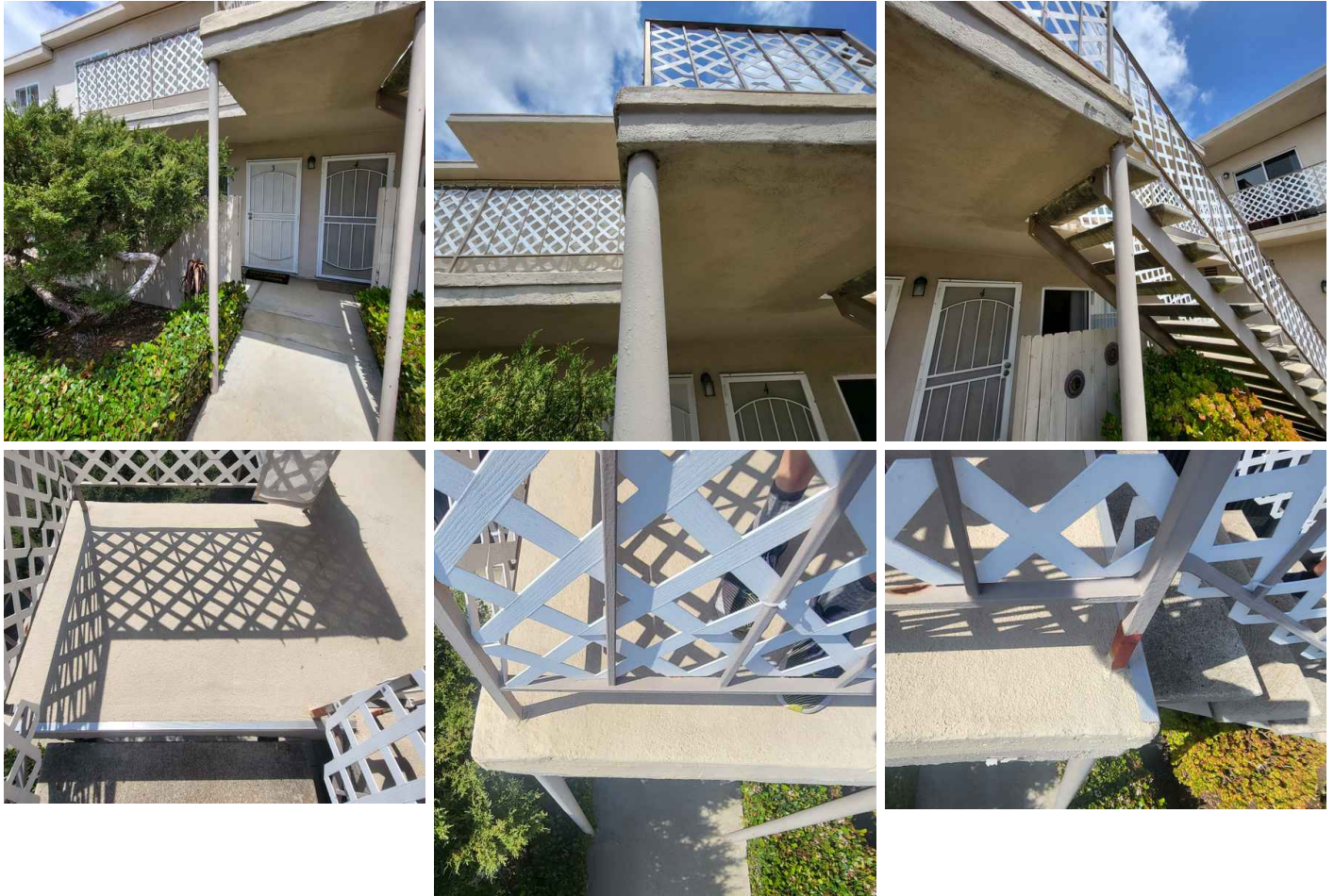
Walkway: Support Material Wood
