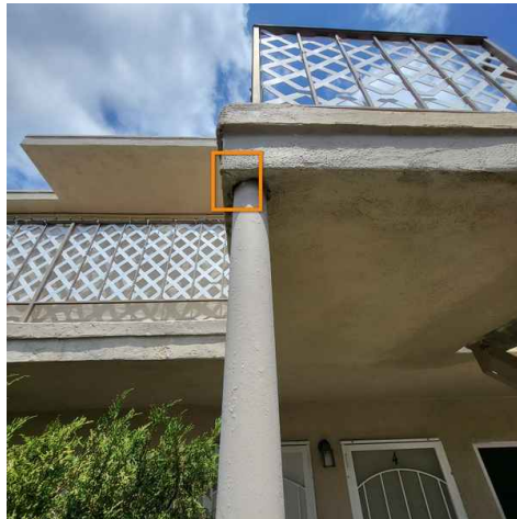
cracking
