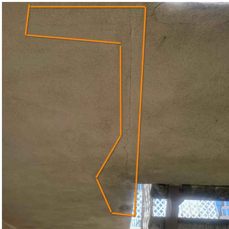
cracking, stained
