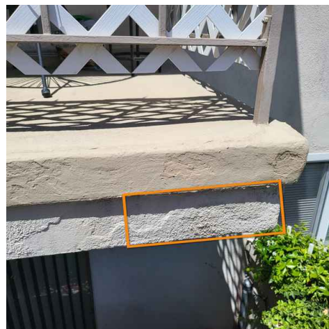
bubbling, efflorescence
