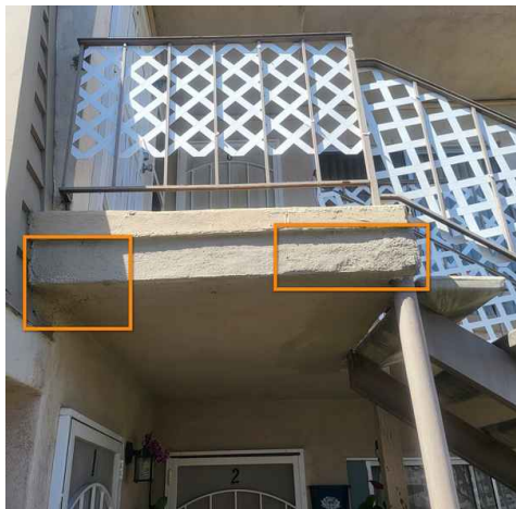
bubbling, efflorescence
