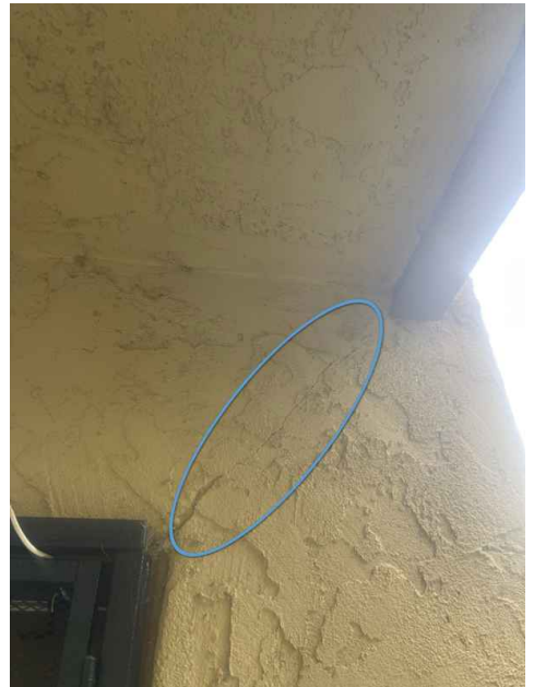
Underside of Entry Structure
