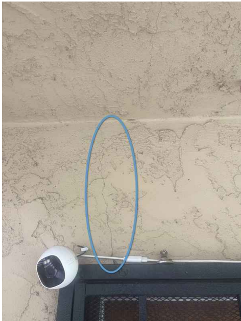
Underside of Entry Structure
