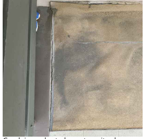
Crack in sealant above termite damage
