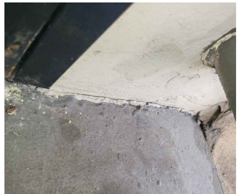
Crack in sealant above termite damage
