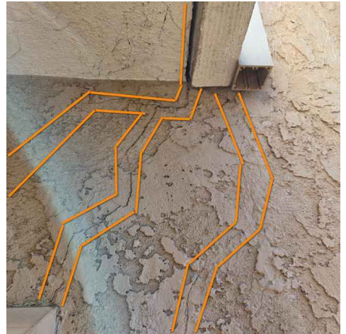
Underside of SE corner of Balcony 4
