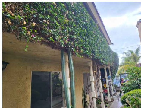
Underside of walkway N view
