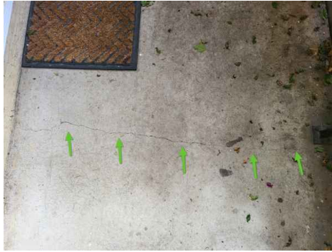
Crack across concrete deck
