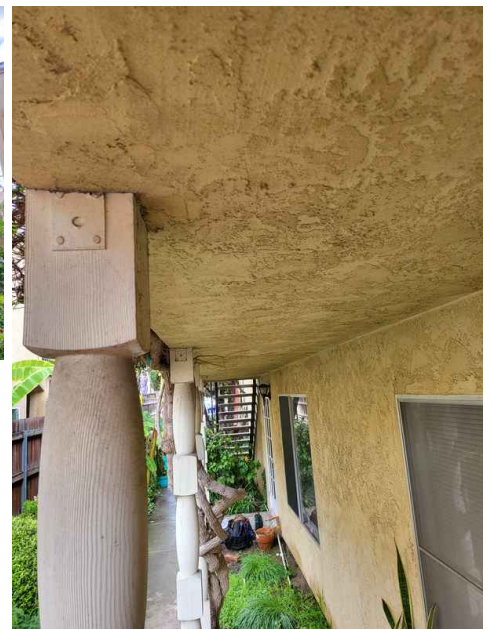
Underside of walkway S view
