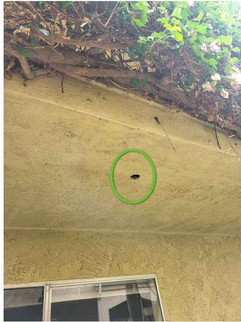
1st borescope inspection
