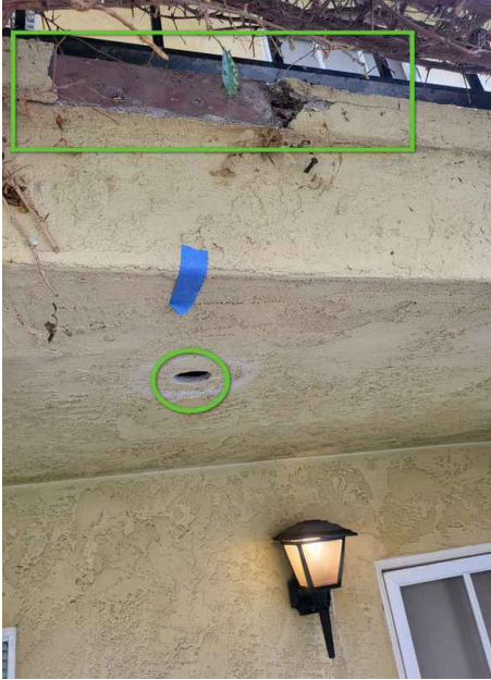
4th borescope hole
