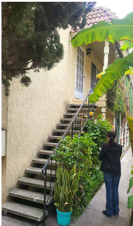
Stairs to walkway
