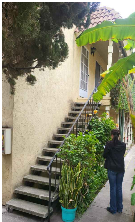
View of stairs and walkway E3s
