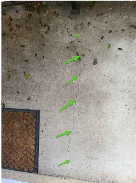
Crack across concrete deck
