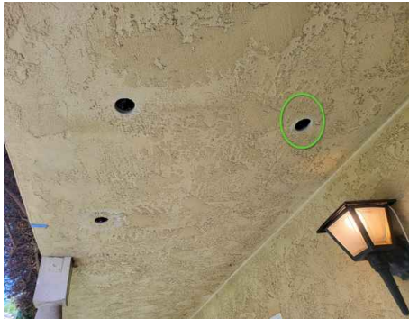
7th borescope hole
