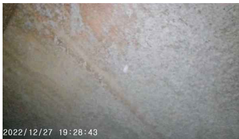
Crack across concrete deck
