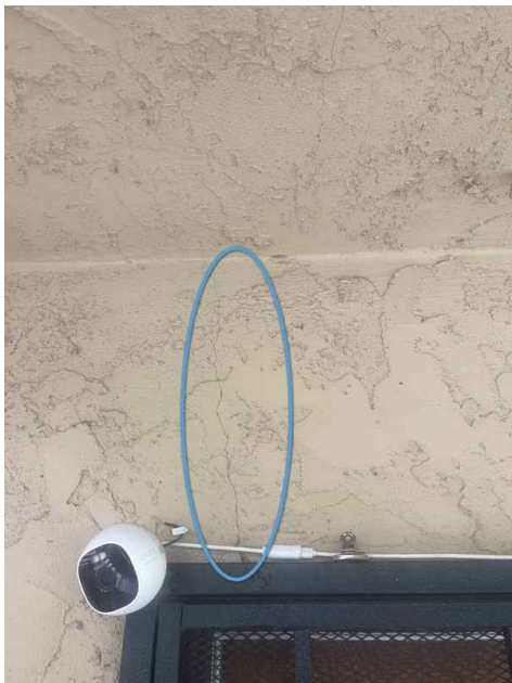
Underside of Entry Structure
