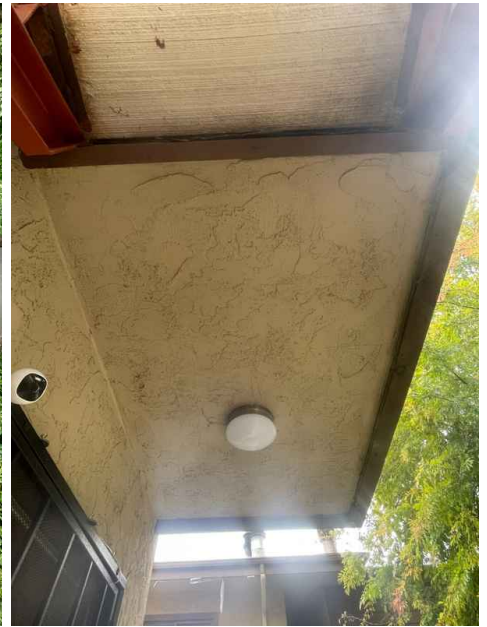
Underside of Entry Structure
