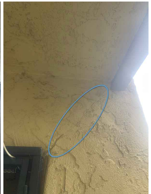
Underside of Entry Structure
