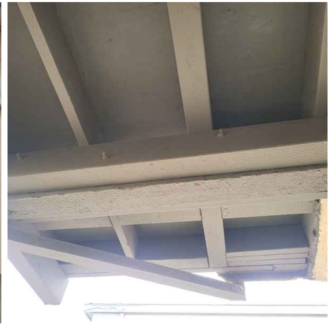
Underside of Landing
