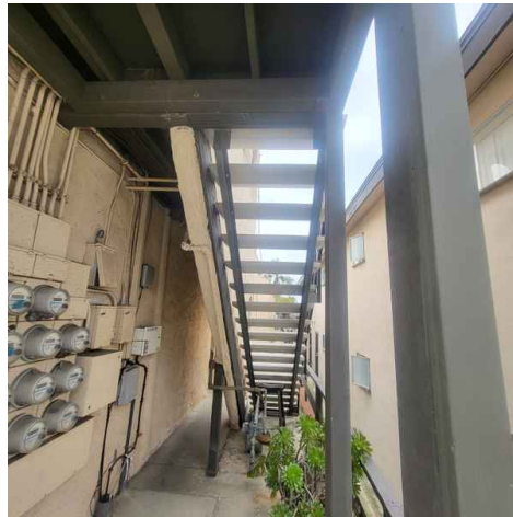
Underside of Landing
