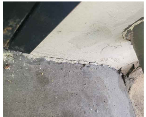
Crack in sealant above termite damage
