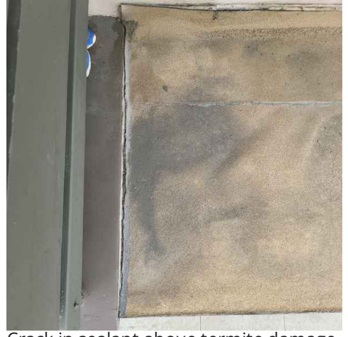
Crack in sealant above termite damage
