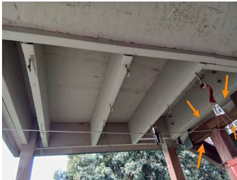
Temporary Support Beam
