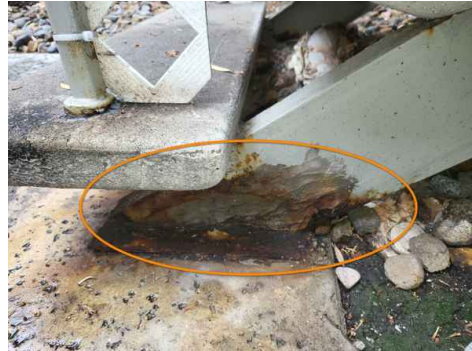
Bottom of stringer
