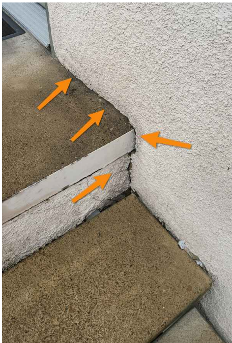
Group 3 E stairway
