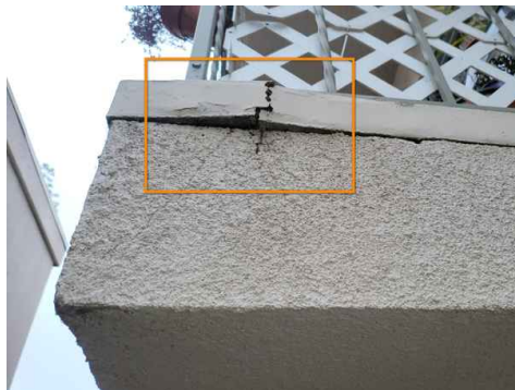
Group 2 Edge Metal N End of Walkway
