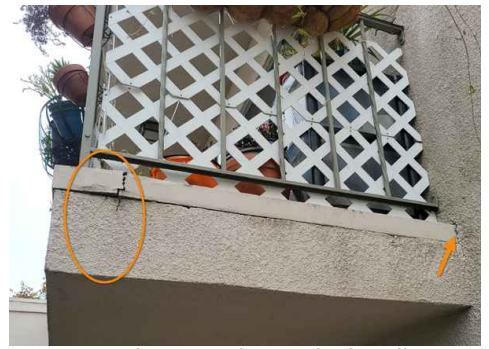
Group 2 Edge Metal N End of Walkway
