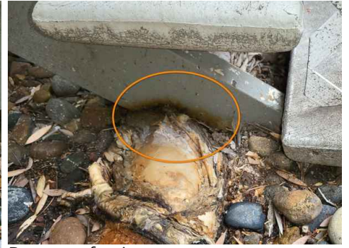
Bottom of stringer
