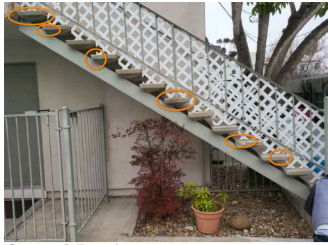
Group 3 E stairway
