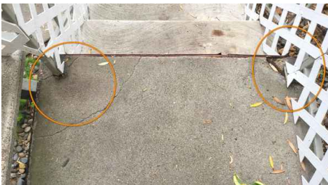
Group 1 Stairway landing
